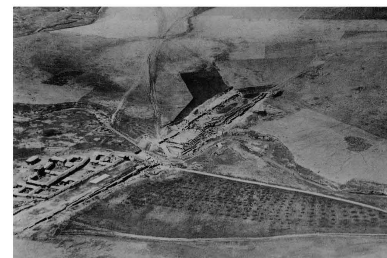
Fig. 3. Excavations at the aqueduct at Jerwan. The aqueduct spanned a wadi (seasonally flowing drainage). The continuation of the canal can be seen as a dark line running toward the top of the image.
